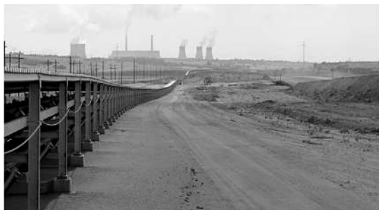
Figure 1: Belt Conveyor KW-05 of the Optimum overland system.
